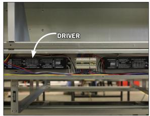
Fig. 7 Electrical raceway
