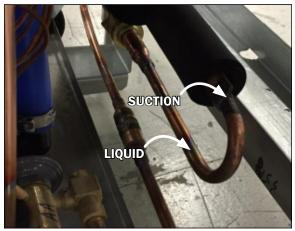
Fig. 5 Refrigeration suction and liquid connections
