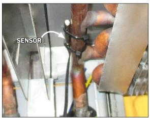
Fig. 4 Gravity coil sensor
